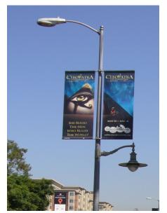
TYPE A: Pedestrian Light Retrofitted to Existing Street Lights (Figure B.1.v)
